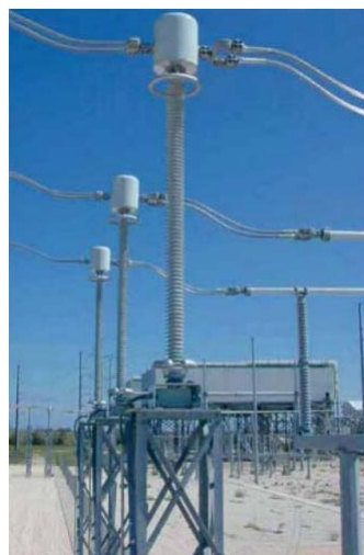
Figure 8 – Installation of a CT with an optical sensor
