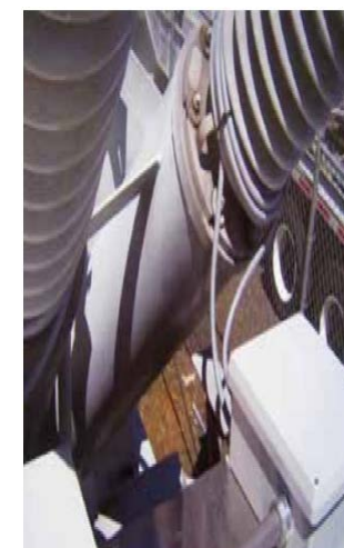
Figure 6 – Alstom COSI-NXCT F3 flexible optical current transformer in a portable substation application
