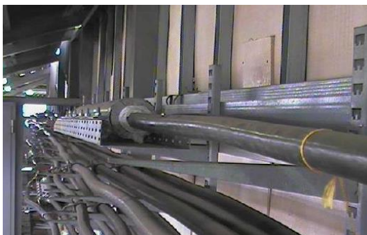
Figure 1. Connection of cable lines with couplings
