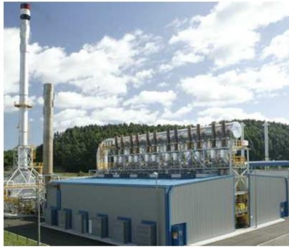
Figure 2.5 – Power plant on converter gas from Aceralia plant
