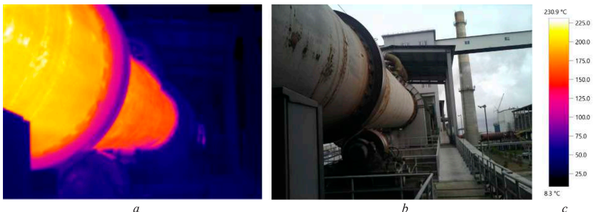
Fig. 1. Thermal fields of the surface of the coke calcination furnace:
